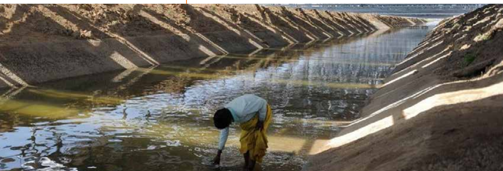
► Gujarat's Canal-Top-Solar panels are suspended on a metal structure over the canal (Credit: Getty Images)
