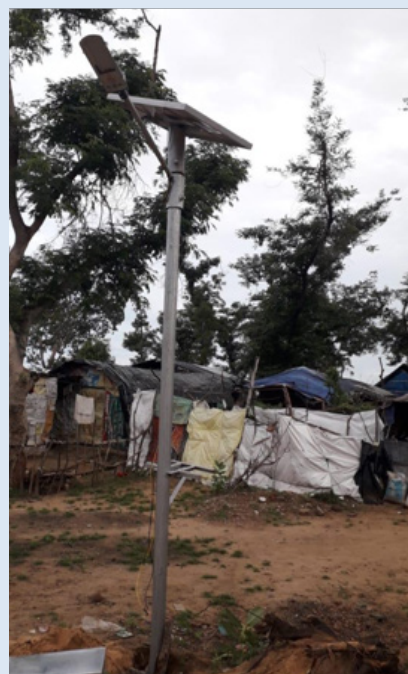
Solar-powered streetlight in Odisha after Cyclone Fani
