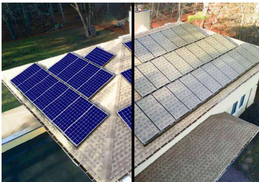
Figure 1: A comparison of a traditional solar panels vs the panels with “solar-skin”
