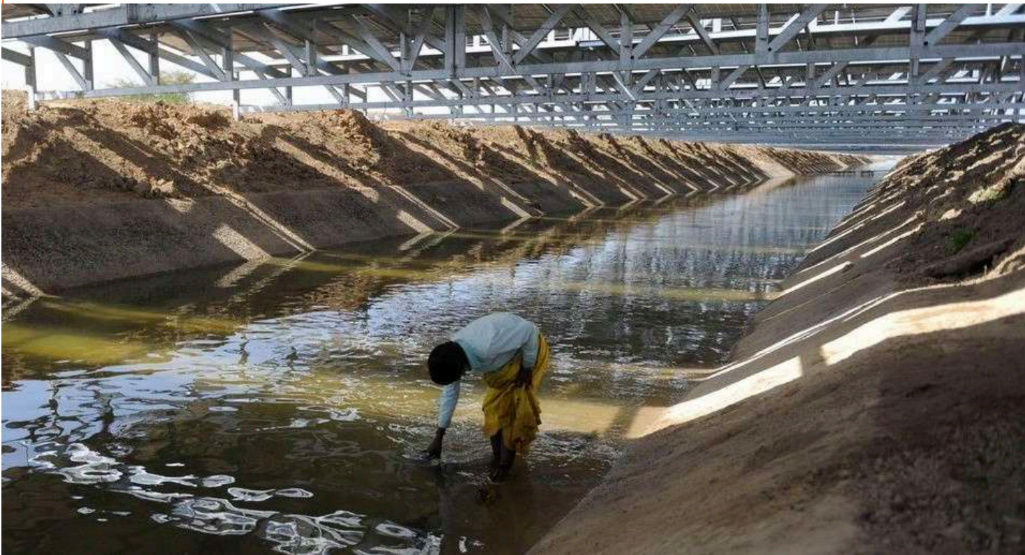
Gujarat's Canal-Top-Solar panels are suspended on a metal structure over the canal
