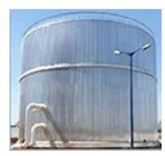
**Figure 3:** Thermal storage tank (using chilled water) for the district cooling system at GIFT City
